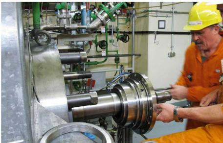
An EagleBurgmann **SHV1/165-E2-Q** mechanical seal is applied as shaft seal on the main feedwater pump at the E.ON Isar I nuclear power plant in Germany. Operating conditions:  $p = 20 \text{ bar}$  (290 PSI);  $t = 185 \text{ }^\circ\text{C}$  (365  $^\circ\text{F}$ );  $n = 5,730 \text{ min}^{-1}$ .
