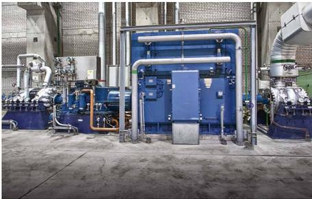
The RWE power plant in Niederaussem, Germany uses a Weller pump in the feedwater circuit. A mechanical seal type **SAPV1/138-E2** along with a **SPF9025/A005-V1** seal supply system is applied. Operating conditions:  $p = 20.2 \dots 27.5 \text{ bar}$  (293 ... 399 PSI);  $t = 177 \text{ }^\circ\text{C} \dots 201 \text{ }^\circ\text{C}$  (351 °F ... 394 °F);  $n = 1,000 \dots 5,100 \text{ min}^{-1}$ .
