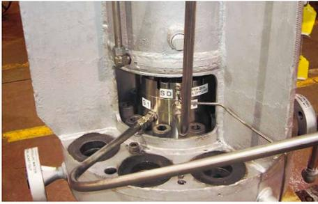
A boiler circulation pump is installed in the feedwater circuit at the municipal power plant in San Antonio, Texas. The pump shaft is sealed by two **SHFV3/125-FTA** mechanical seals. Operating conditions:  $p = 170 \text{ bar}$  (2,465 PSI);  $t = 340 \text{ }^\circ\text{C}$  (644 °F);  $n = 1,800 \text{ min}^{-1}$ .
