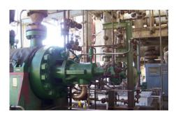
**H75KF-D1/130** back-to-back dual seals with supply system **SP09030/M012-D1** to API 682 Plan 53 have been successfully sealing the shafts of Pacific between bearing pumps since 2004. The system is located in the CRP refinery of Petroleos De Venezuela S.A. Operating conditions: p = 4 barg (58 PSIG); t = 200 °C (392 °F); n = 3,600 min<sup>-1</sup>; d1 = 104.1 mm (4"). Media: naphtha, gasoil + 3 % H<sub>o</sub>S.
