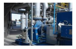
Stripper reflux pumps within the naptha hydro treater unit of the ENOC refinery in Dubai are fitted with EagleBurgmann **H75VKS20/105** mechanical seals and supplied to API 682 Plan 11. Operating conditions:  $p=11.77 \text{ bar } (25 \text{ PSI}); t=43 \text{ °C } (109 \text{ °F}); \\ n=1,485 \text{ min}^1; d1=80 \text{ mm } (3.15").$  Media: hydrocarbons.
