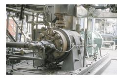
EagleBurgmann **MFLWT80S3/90** sealing Byron Jackson pumps supplied to API 682 Plan 02 + 54 by an EagleBurgmann **SPA 3020/A22** supply system. Operating conditions:  $t = 332 \,^{\circ}\text{C}$  (630  $^{\circ}\text{F}$ ); p = 8.5 bar (123 PSI). Medium: residual oil.
