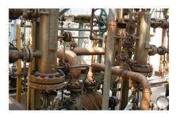
The shafts of KEPL pumps of Chennai Petroleum Corporation Ltd. in India are reliably sealed by EagleBurgmann metal bellows seals type MFLWT80/90 and MFL65F/85. Operating conditions:  $p = 16.08 \dots 19.93$  bar (233 ... 289 PSI);  $t = 238 \, ^{\circ}\text{C} \dots 263 \, ^{\circ}\text{C} (460 \, ^{\circ}\text{F} \dots 505 \, ^{\circ}\text{F});$  $n = 2,955 \text{ min}^{-1}$ ; d1 = 80 mm (3.15"). Media: hydrocarbons.
