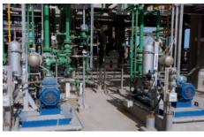
In the ENOC refinery in Dubai, U.A.E., LPG pumps are sealed by EagleBurgmann **H75VKS20/85** dual tandem face-to-face mechanical seals. Applied API piping plans: 11 + 53B. Operating conditions: p = 17.75 bar (257 PSI); t = 43 °C (109 °F); t = 2.950 min<sup>-1</sup>; t = 60 mm (2.36"). Media: hydrocarbons.
