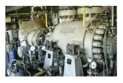
A high pressure dry gas seal EagleBurgmann type PDGS2.1/130 seals a Bhel compressor in the hydrocracker unit of the Panipat refinery in India. Operating conditions: p = ... 179 bar (2596 PSI);  $t = 160 \,^{\circ}\text{C} (320 \,^{\circ}\text{F}); d1 = 112 \,^{\circ}\text{mm} (4.41").$ Media: H2 + CH4, N2.
