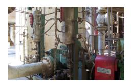
Since 2001, PDVSA (Petroleos de Venezuela) has been using EagleBurgmann seals type H75K/110 with supply system **TS6050** to API 682 Plan 52 in a Sulzer between bearings pump. Operating conditions: p = ... 4 bar (58 PSI); t = 52 °C  $(126 \, ^{\circ}F); n = 3,560 \, \text{min}^{-1}; d1 = 80 \, \text{mm} (3.15").$ Media: aromatic hydrocarbons.
