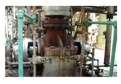
EagleBurgmann **LL9DTUU** dual mechanical seals are applied to seal a Sulzer pump of a catalytic cracking unit operated by Chennai Petroleum Corporation Ltd. in India. Operating conditions: p = ... 13.73 bar (199 PSI);  $t = 40 \, ^{\circ}\text{C} (104 \, ^{\circ}\text{F}); n = 2,965 \, \text{min}^{-1};$ d1 = 70 mm (2.7"). Media: hydrocarbons.
