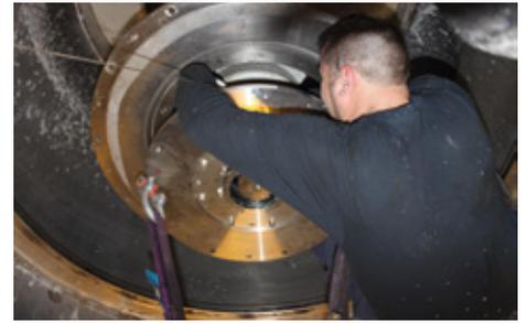
A **Pulpex-S/135-00** is installed in a sorter at the Sappi paper mill in Lanaken/Belgium. The mechanical seal runs in a continuous process in pulp preparation. Operating conditions:  $p = 3.5 \text{ bar (51 PSI)}$ ,  $t = 80 \text{ }^\circ\text{C (176 }^\circ\text{F)}$ ,  $n = 800 \text{ min}^{-1}$ . Medium: pulp.
