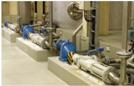
At Iggesund Paperboard, Workington, UK, eccentric screw pumps with MG1S50 type cartridge seals are operating reliably in the coating plant. Medium: Coating color,  $p_3 = 4$  bar (58 PSI),  $t_3 = 40 \text{ }^\circ\text{C}$  (104  $^\circ\text{F}$ ),  $n = 850 \text{ min}^{-1}$ .
