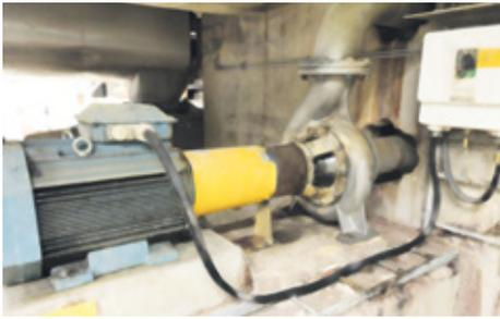
**MG1S14** type elastomer bellows seals are supplied as standard cartridge and also fit in ABS Scanpump pumps and Sulzer APP pumps. Alone more than 40 seals are being applied successfully at the Stora Enso Kvarnsveden/Sweden paper mill. Operating conditions:  $p = 8 \dots \text{max. } 10 \text{ bar (116 ... 145 PSI max.)}$ ,  $t = 60 \text{ }^\circ\text{C (140 }^\circ\text{F)}$ ,  $n = 1,490 \text{ min}^{-1}$ .
